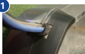
Handrail entry safety protection Protection against risk of foreign matters being jammed into handrail entry
